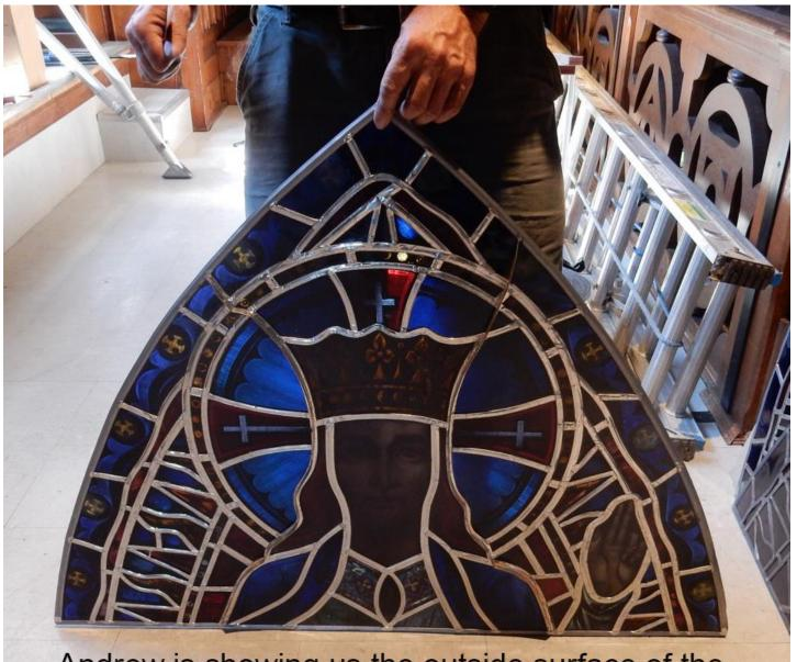
Andrew is showing us the outside surface of the panel. The lead strips (cames) on the outside are reinforced by tin, which is shiny. The tin makes the window more rigid and less likely to buckle. Also, you get a sense of the size of the panel.
