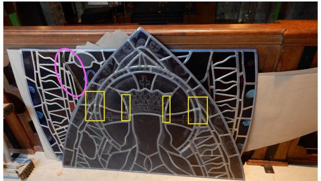
Panels waiting to be installed. The panel of Christ's head and shoulders is facing with the interior surface showing. The yellow rectangles highlight tie wires that will attach to window support rods. In back, on the outward facing side, shiny tin cames are visible on a different panel. The pink ellipse shows one of the new support braces that follow some of the cames on the exterior side of the panels.
